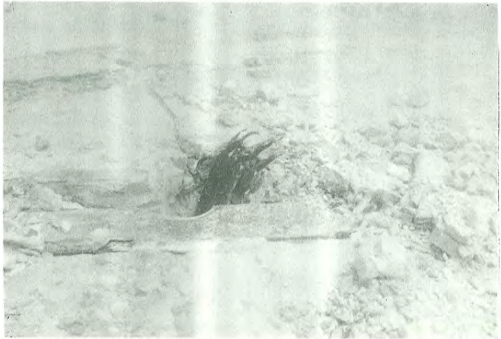
Figure 5.2 Part of grouted stone bed with protruding ends of a ruptured rock anchor tendon
